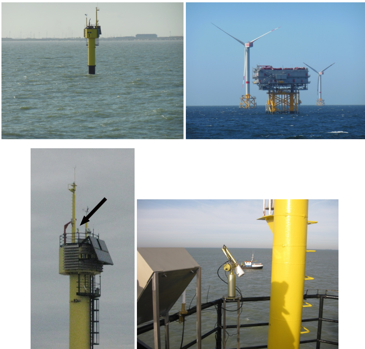
Figure 2 Photos of the platforms used for the new Belgian AERONET-OC sites: (top-left) Zeebrugge-MOW1 measurement platform, (top-right) Thornton-CPOWER offshore transformer platform, (bottom-left) SeaPRISM instrument location and (bottom-right) SeaPRISM instrument as installed at Zeebrugge-MOW1.
